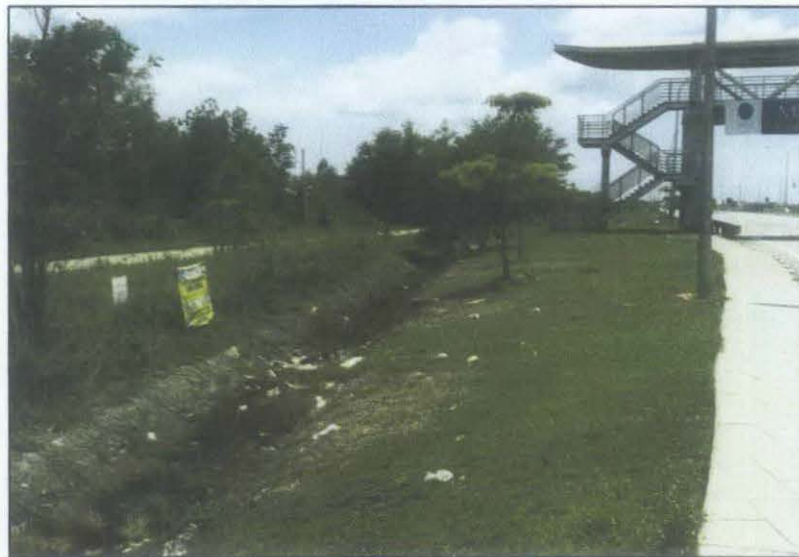
Figure 3.2: Drainage in front of Universiti Teknologi Petronas
