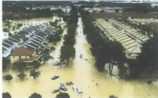
Figure 1.2: The picture shows a section of Taman Tun Dr Ismail Jaya in Shah Alam, Selangor, submerged in floodwaters (The Star - Residents rudely awakened by floodwaters, February 27, 2006).
