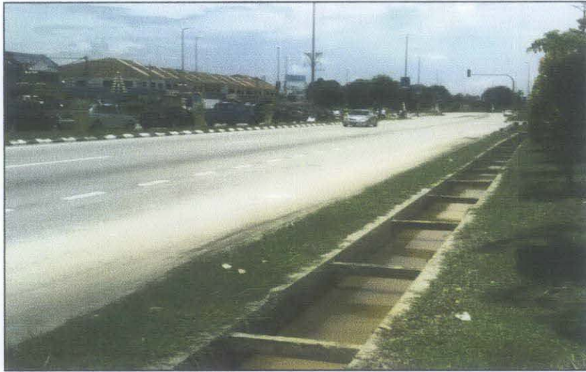
Figure 3.3: Drainage along Taman Maju
