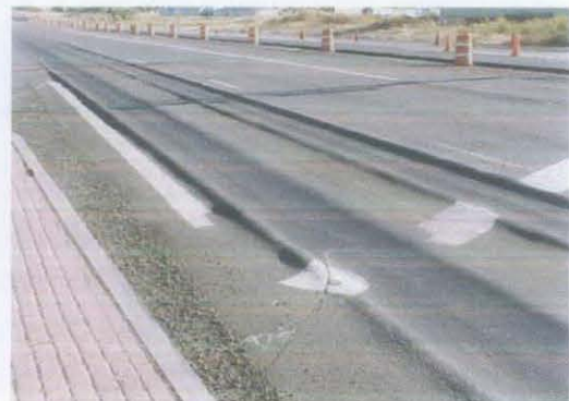
Figure 1.5: Rutting Pavement
