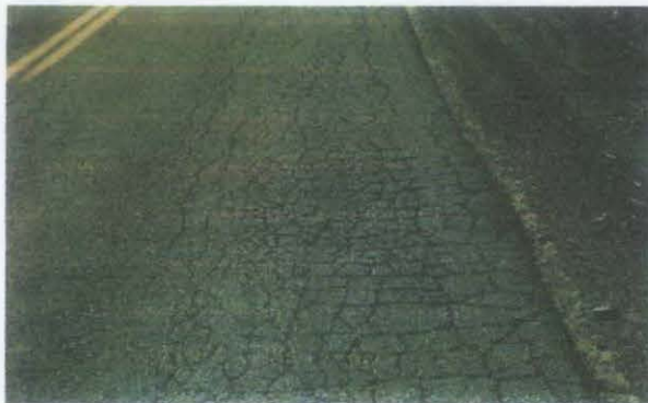
Figure 1.4: Cracking Pavement
