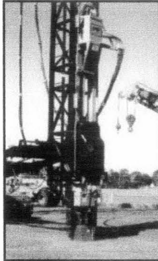
Figure 2.10: Hydraulic hammers
