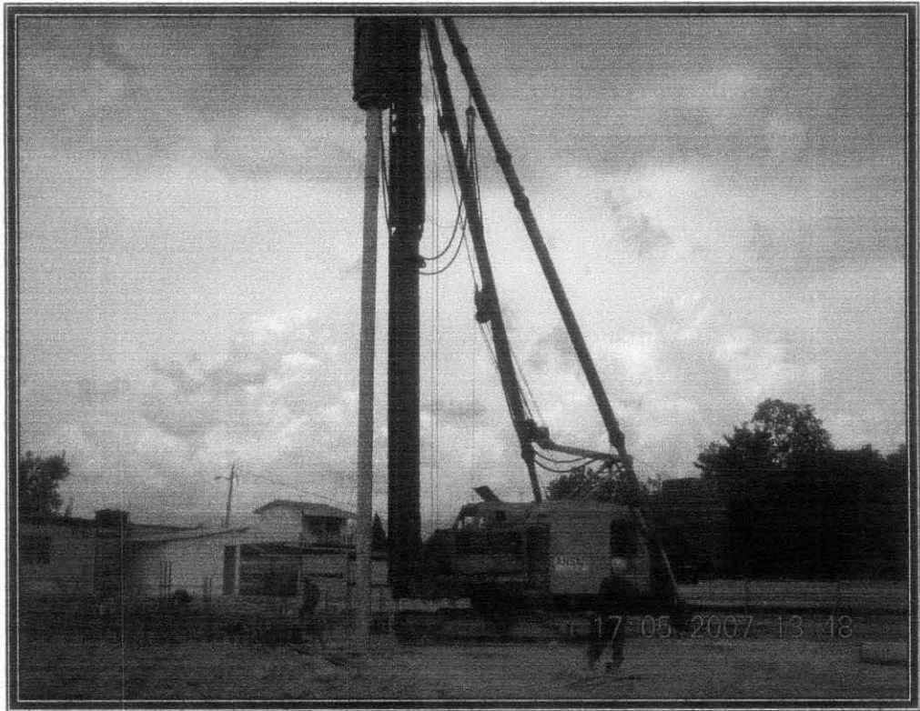
Figure 2.2: Hydraulic Hammer Junttan 7.0 ton
