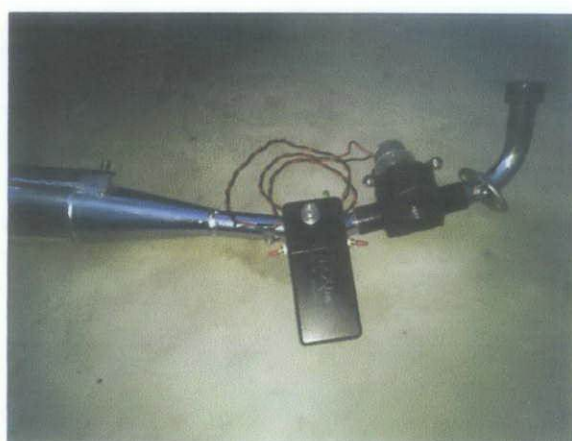
Figure 40: Electrical circuit connected to the generator.
