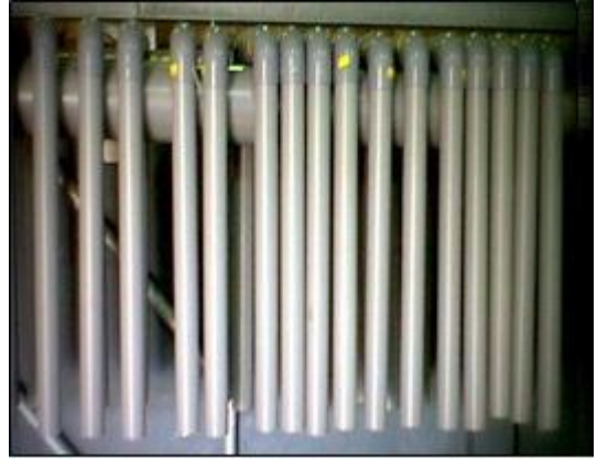
Figure 8: Hanging the U-Shaped Vertical Pipe onto the Rectangular Pipe
