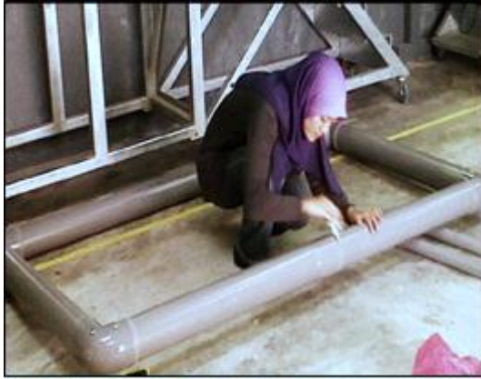
Figure 7: Fabrication of Rectangular Pipe (Top part)
