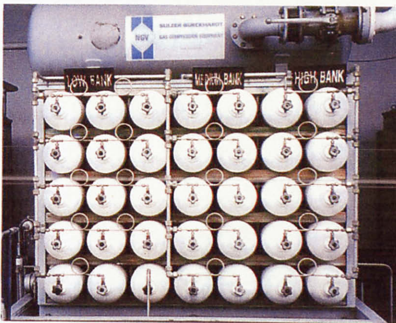
Figure 2.5: A typical NGV storage cascade [2]
