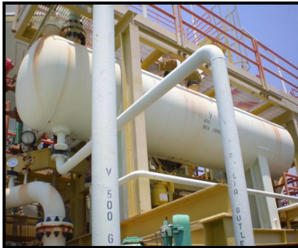
Figure 1.2: Horizontal Separator. Type of vessel that can be grinded.
