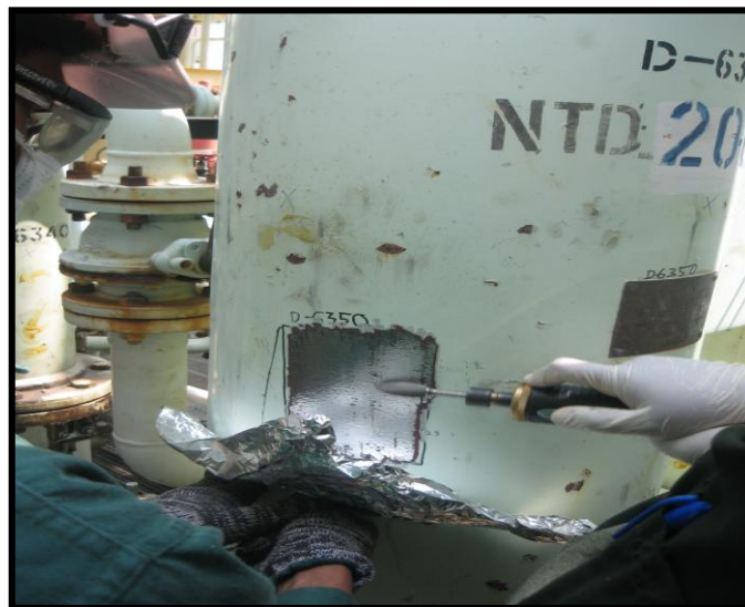
Figure 4.1: A conventional manner of grinding process. This process needs 2 people to perform the micro grinding process. One person hold 2 rounded magnet below the aluminium foil whilst other person operates the grinder machine.
