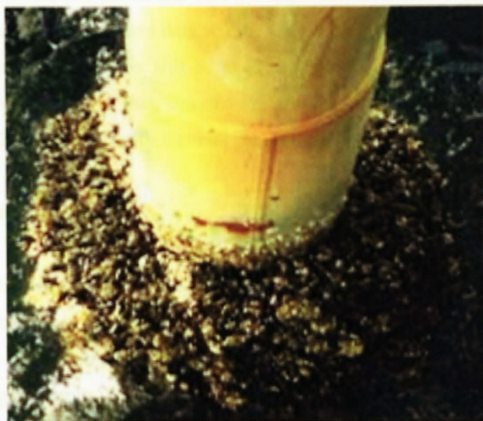
Figure 2.4: Example of marine growth at the platform
