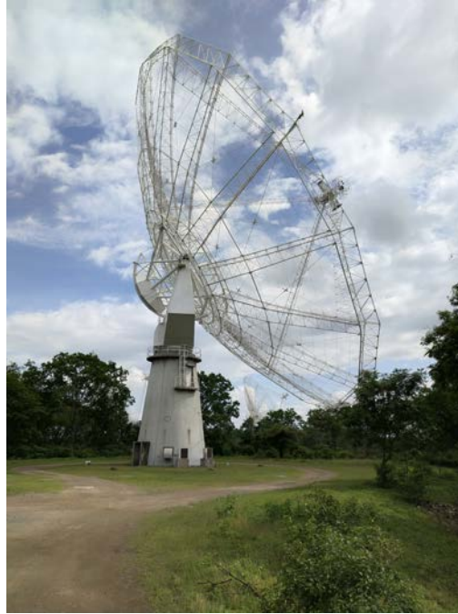
Figure 2.16: The light-weight wire mesh is used to lower the wind forces and to cut the cost on building the array. This is the C02 antenna picture taken by the author in the central square with two other antennas at the background (C03 & C04).
