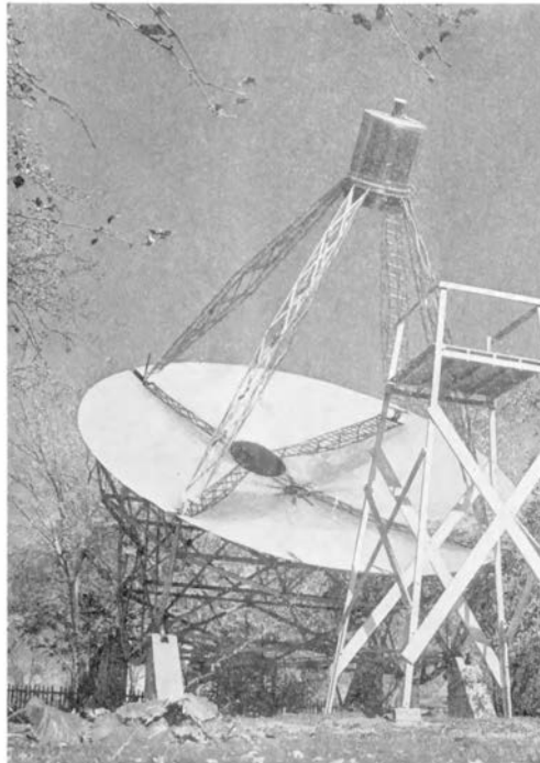
Figure 2.2: The 9 meter parabolic reflector telescope built in Wheaton, Illinois for the first sky survey at 160 MHz (Reber, 1944).
