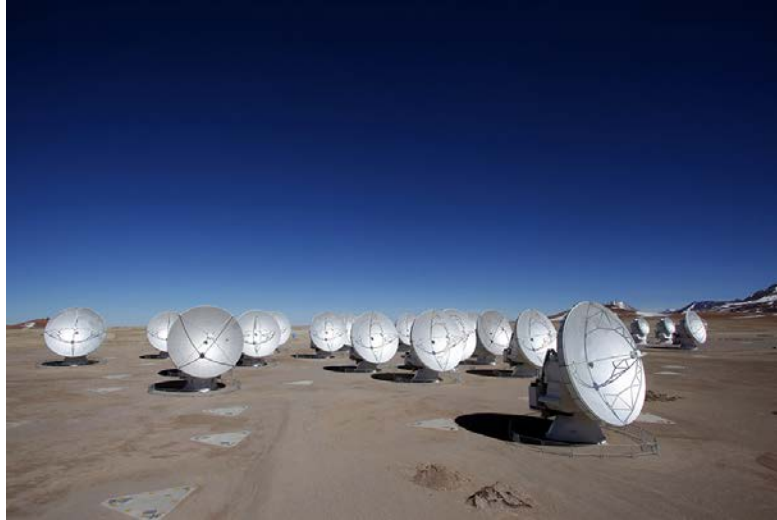
Figure 2.12: ALMA antennas at the Array Operation Site (AOS) located in the Central Cluster. There are a total of 118 foundations where the antennas are located, extended over 32 km in diameter for 66 antennas. Notice that the highly polished reflective surface that enable the sub-mm observation. Image Credit: Carlos Padilla - AUI/NRAO.
