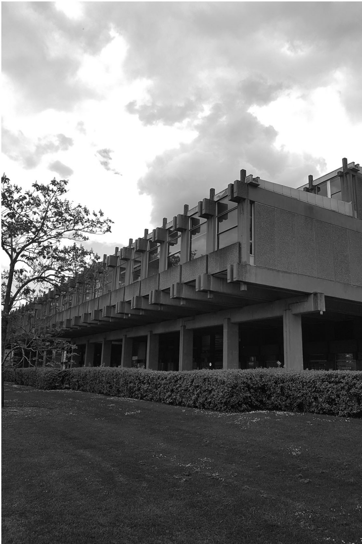
Figure 1. The external envelope of the URS building.
