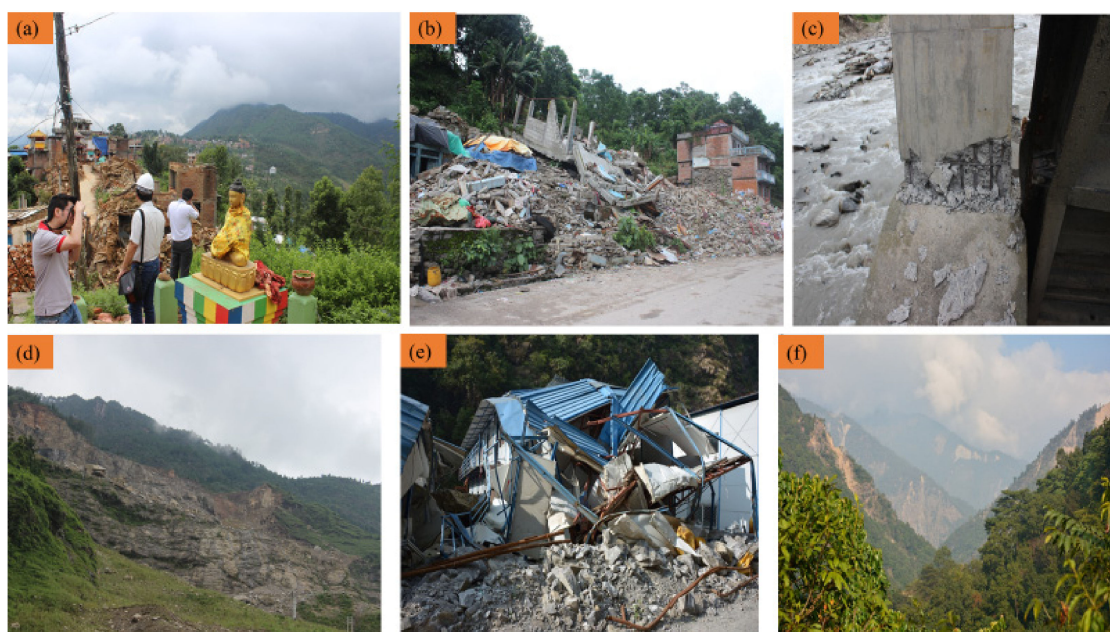
Figure 15. (a) Damaged settlement across a ridgeline in Sindhupalchowk district, (b) destroyed settlement along the Arniko Highway in Sunkoshi–Bhotekoshi watershed, (c) damaged pier of the Sunkoshi hydropower project reservoir site, (d) reactivated Jure landslide due to the earthquake, (e) damage to water supply infrastructure, (f) landslides triggered in the mountains across the Bhotekoshi–Sunkoshi watershed.
