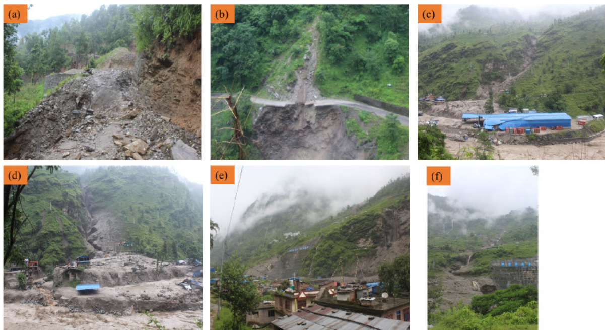
Figure 13. (a) Rural road section wiped out by debris flow, (b) highway section damaged by debris flow, (c) damage to warehouse, (d) completely destroyed Jambu neighborhood by debris flow, (e) damage to Middle Bhotekoshi Hydropower Project, (f) widening of debris flow along the gorge.
