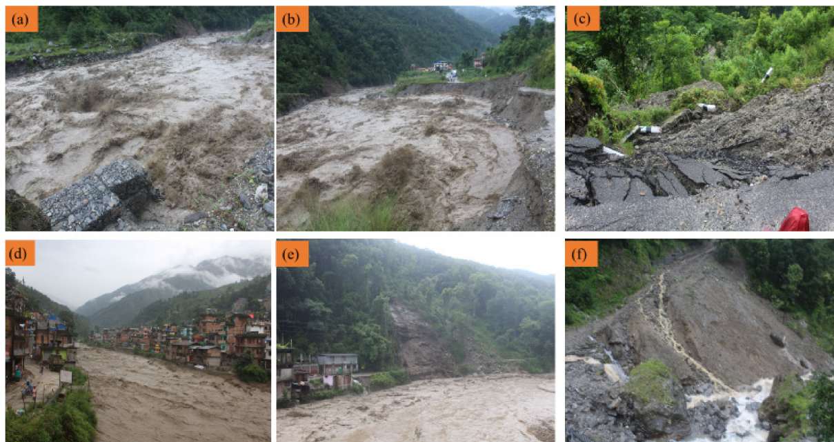
Figure 12. Effects of flooding and debris flow: (a) toe cutting and subsequent damage to protection structure by Sunkoshi River, (b) mass movement and slope failure due to toe bank erosion, (c) highway section damaged due to debris flow, (d) flooding in Bahrabise neighborhood, (e) obstructed road section due to slope failure, (f) slope failure across a gorge.
