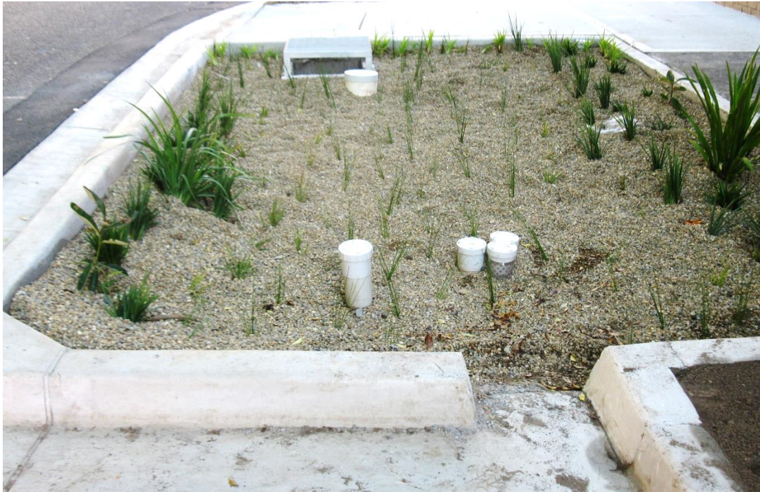
Figure 5: Field stormwater biofilter system, operated by the City of Sydney (photo courtesy of Chris Derry)
