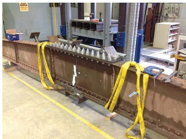
Figure 8: Completed retrofit for RMS 120-year-old girder.
