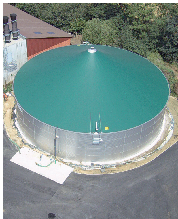
Image 10: Covered storage of liquid manure (Manure Measure 1) avoids contact with air and reduces both ammonia and odour emissions, while the containment provided also avoids aquatic nitrogen losses (photograph: © Stallkamp).
