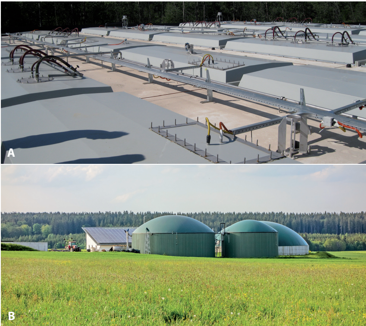
Image 12: Two examples of on-farm anaerobic digestion facilities, which provide an opportunity to recover biogas and nitrogen rich digestate (Manure Measure 11). The approach should be integrated with low emission spreading, ammonia stripping or other nutrient recovery to avoid subsequent ammonia losses. (A, Digestion for a pig farm Russia, photograph © Sergei Lukin; B, System combined with photovoltaics in Germany, photograph © Shutterstock, www.shutterstock.com, ID: 430844485).
