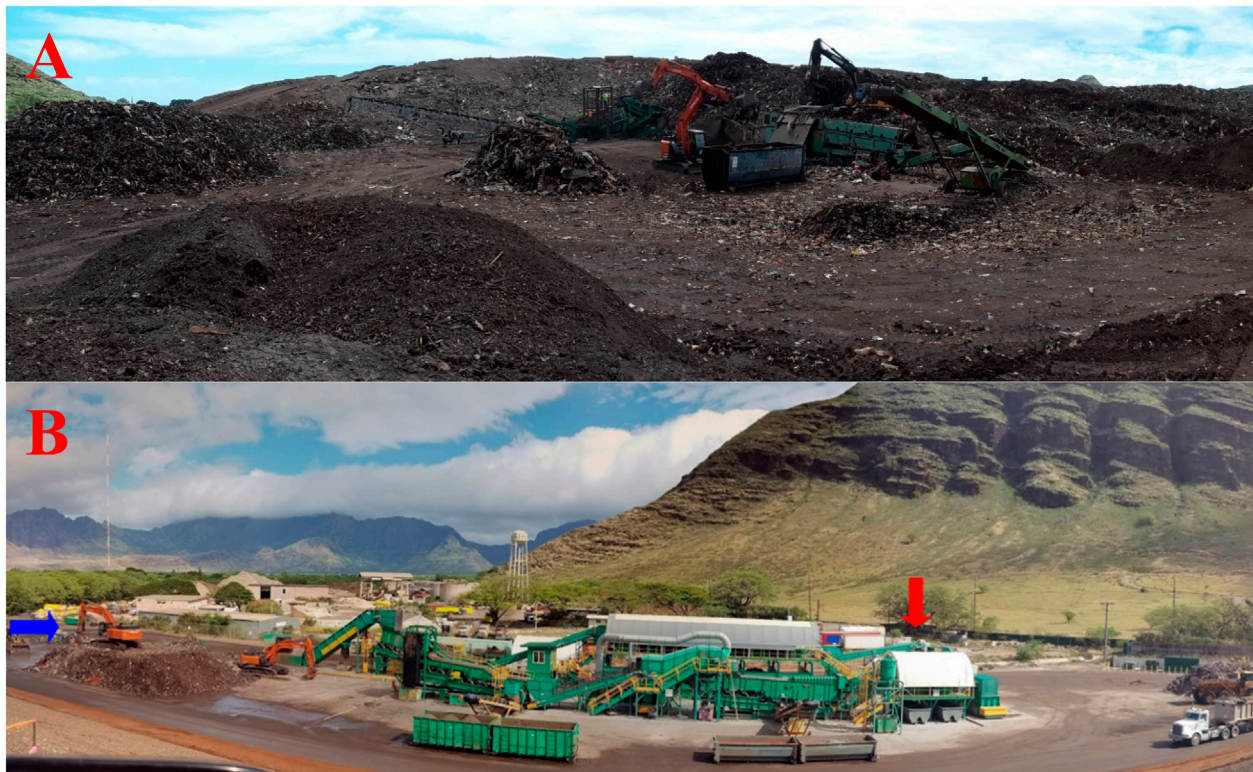
FIGURE 1 | CDWDF materials (A) mining and (B) processing at PVT Land Company (blue arrow: CDWDF intake, red arrow: CDWDF sampling position).
