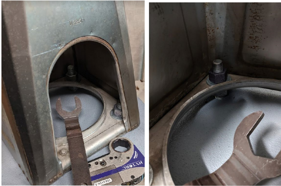
Figure 2.1. Exterior of light pole base (left) and Interior of base (right)
