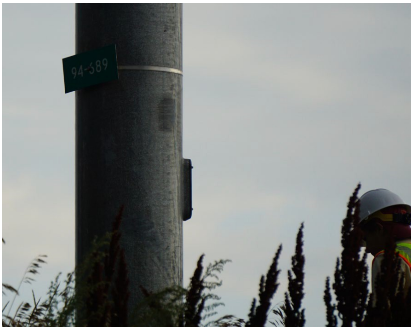
Figure 2.2. Inspection of full truss OH I94-689 sign
