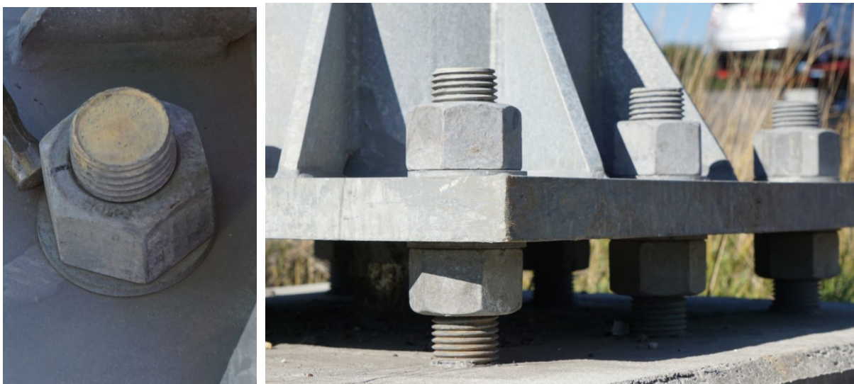
Figure 2.6. Turn-of-nut marks on nut (left) and baseplate of OH I94-688 (right)
