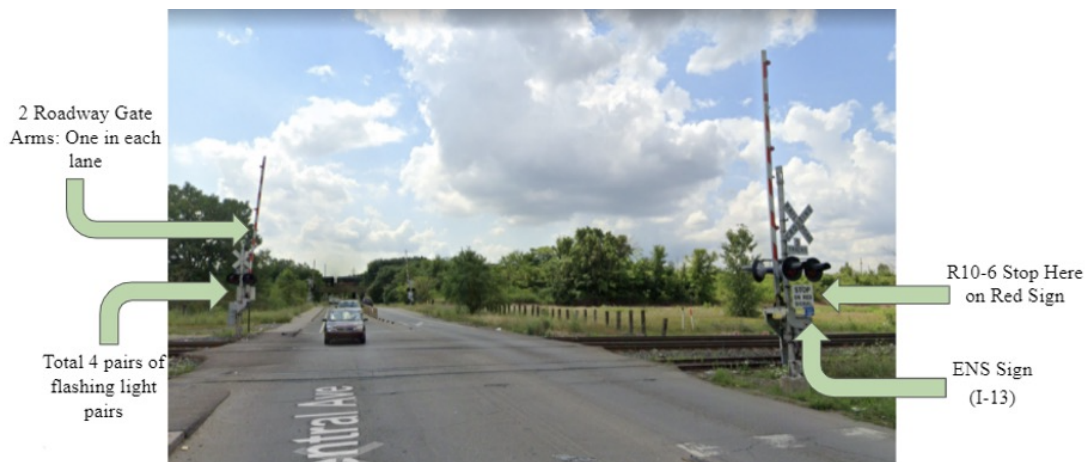
Figure 11: Existing Warning Devices for Central Ave
