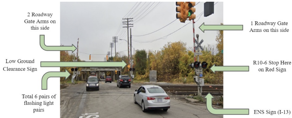
Figure 15: Existing Warning Devices for Lonyo Avenue
