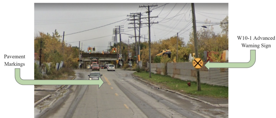
Figure 14: Signage for Lonyo Avenue
