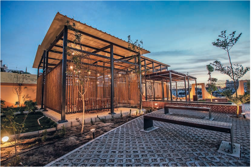
Figure 2. Pavilion rope partitions and surrounding permeable paving/pervious surfaces. Source: © Takween Integrated Community Development 2021.
