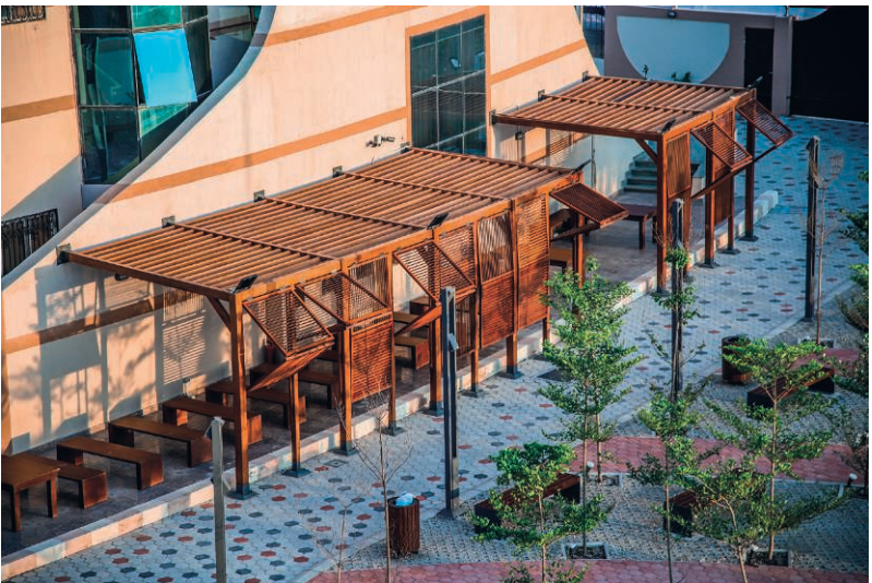
Figure 3. Reading area designed with operable wooden louvres. Source: © Takween Integrated Community Development 2021.
