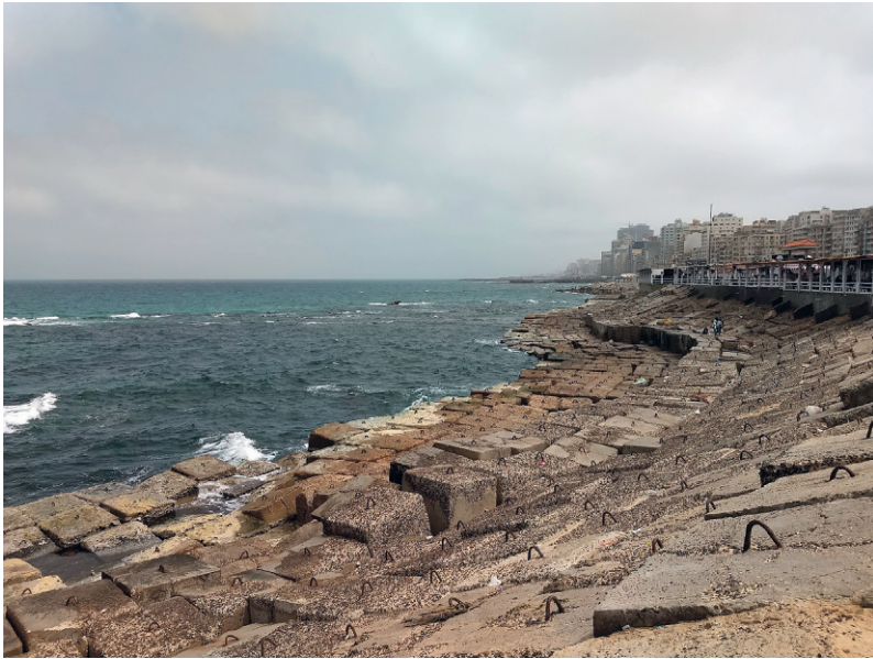
Figures 2b. Coastal defence structures: concrete blocks in Alexandria. Source: F. Bonnefoi, March and April 2021.
