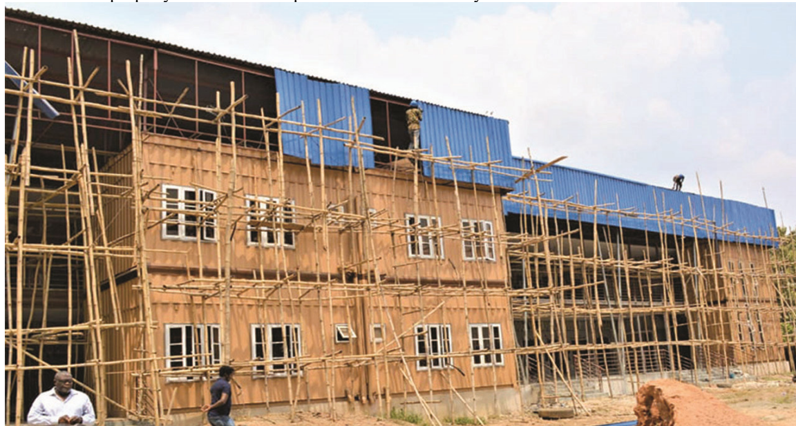
Figure 2: Ongoing Modular 12 classroom block (Nwannekanma 2022)
