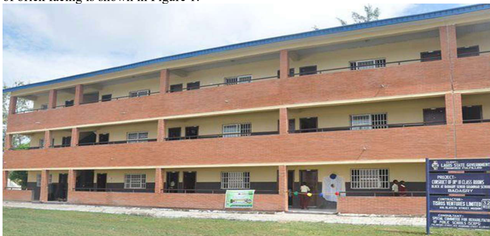
Figure 1: Brick Facing on a School Building (Nwannekanma, 2021)
