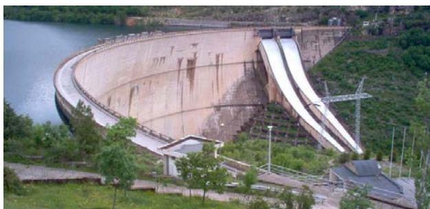
Figure 1. Hydroelectric power station "Trebinje 1", "Grancarevo" dam
