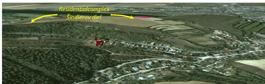
Figure 5.46: The Šindlerov diel residential complex will not be visible from the P7 observation point, the observed objects will be covered by a visual barrier – a relief. (Ortophotomap ©Eurosense, s.r.o.). Adapted from Pauditšová (2015).
