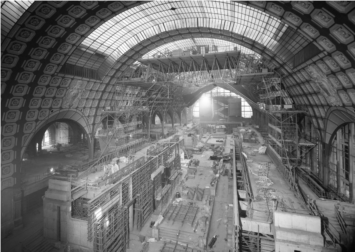
Fig.50 | Construction of Museum (Musée d'Orsay DR Archive, 1984)
