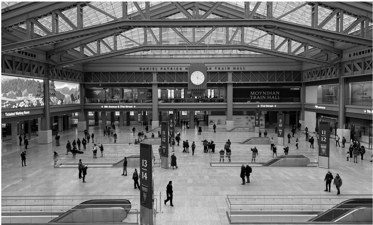
Fig.16 | “Modern” Penn Railway Station (Kauzlarich, 2021)
