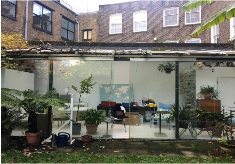
Figure 30: Conservatory within a domestic building
