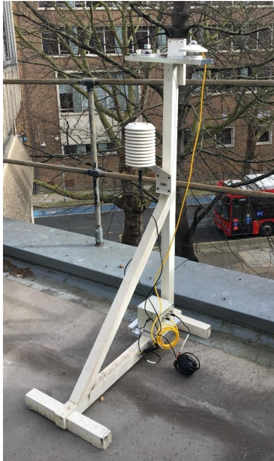
Figure 59: External weather station including a CMP 3 pyranometer, a SKL 310 pyranometer and a rht + probe fitted inside a radiation screen. All of the sensors are connected to DATAHOG2 to enable the saving of the captured data.
