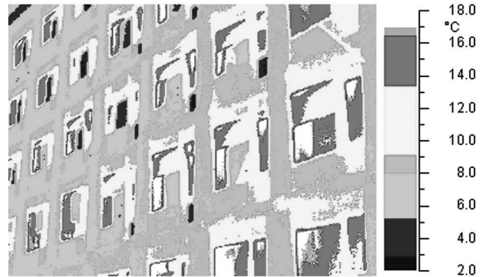
Figure 2. Thermographic survey: building main facade.
