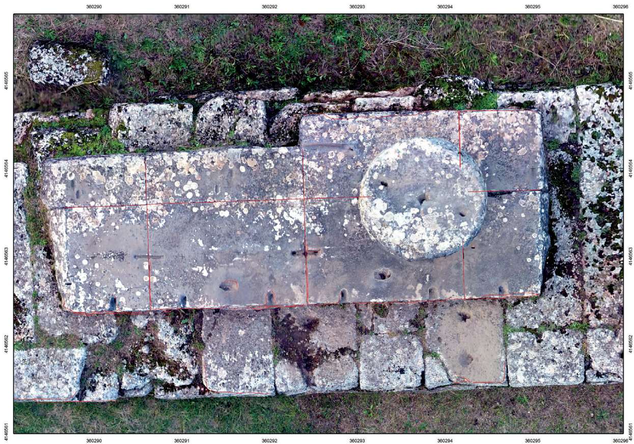
Figure 4. Detail of the south flank of the temple of Athena Alea. The marble euthyteria is on top of the foundation conglomerate blocks, and the column drum is not in situ . The red lines are part of the 3D total station drawing (J. Pakkanen).
