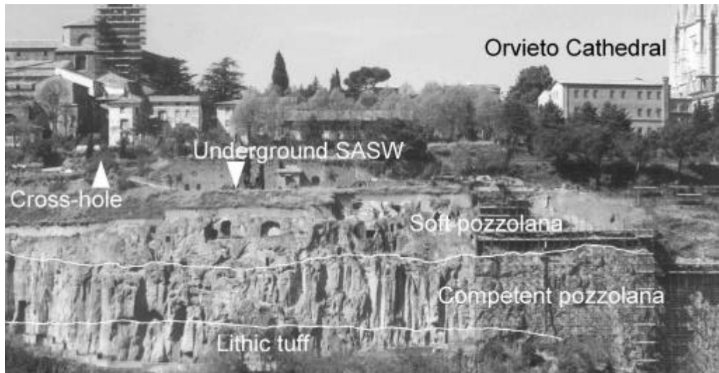
Figure 1. View of the investigation site at the edge of the southern cliff.
