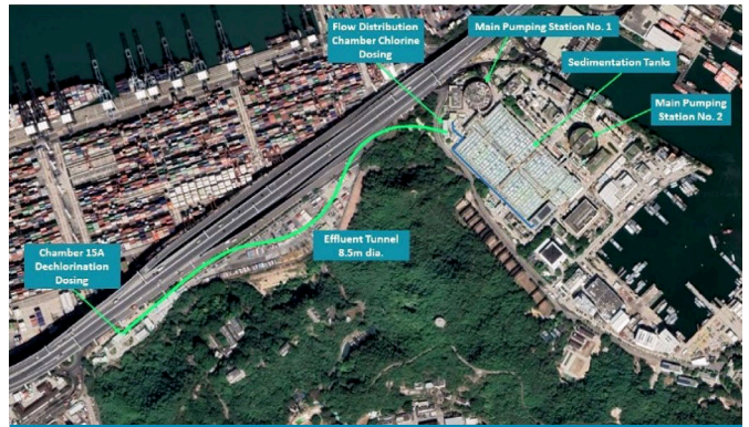
Figure 2 | Chlorine disinfection facilities in the Stonecutters Island Sewage Treatment Works (SCISTW) of HATS (top view).
