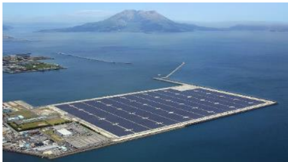
Figure 30a. The ‘Floating’ solar power plant in Kagoshima Bay, Japan can be considered as a good example for saving space. The panels over water have a cooler temperature which makes them more efficient. Finally the blue colour of the panels matches with the blue of the water, hence the panels do not disturb aesthetically. (Photo: © KYOCERA Corporation)
