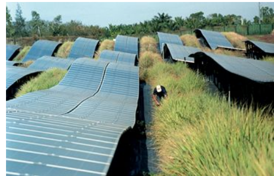
Figure 25d. Type b) Agrinerie® (2.1 MWp), La Reunion (FR). It combines energy generation from PV and lemon grass production. This dual land use design pattern enabled the developers to get the approval for the realization of a system, since in French overseas islands it is not allowed to build on ground PV, because of land and landscape protection rules. (Photo: Akuo Energy)
