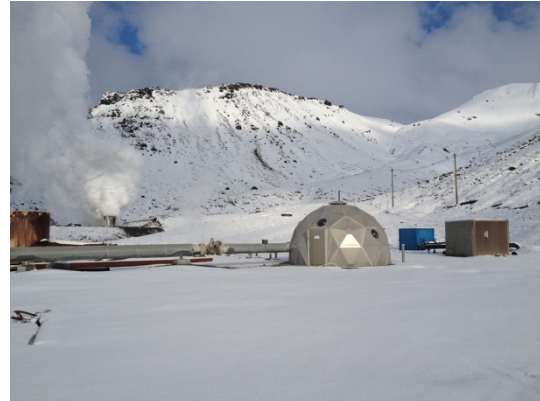
Figure 22b. Geothermal energy plant in Hengill, Southwest Iceland (Photo: David Ostman 2017)
