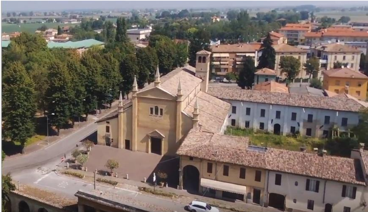
Fig. 1: Aerial photo of the complex.
