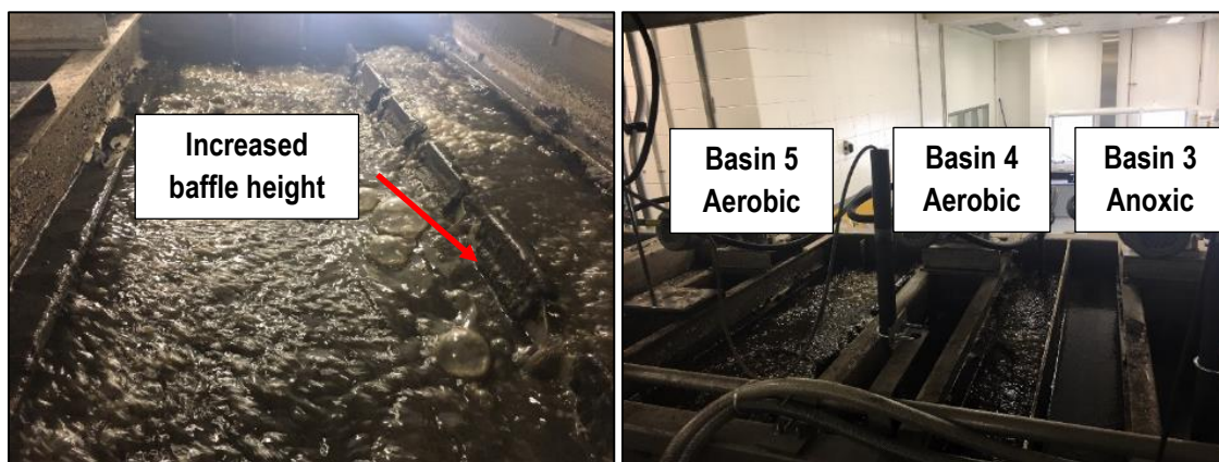
Figure 6.3 The Increased Baffle Height and Flow from 4 th to 5 th Basin
