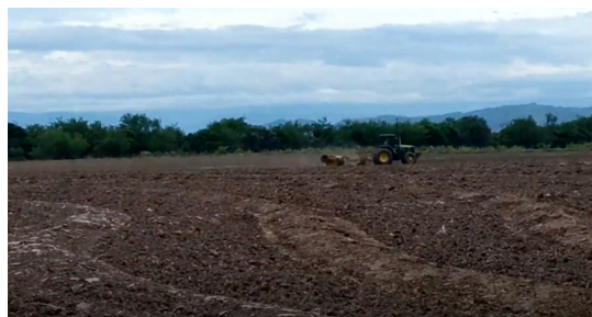
Levees construction using a ridge plough
