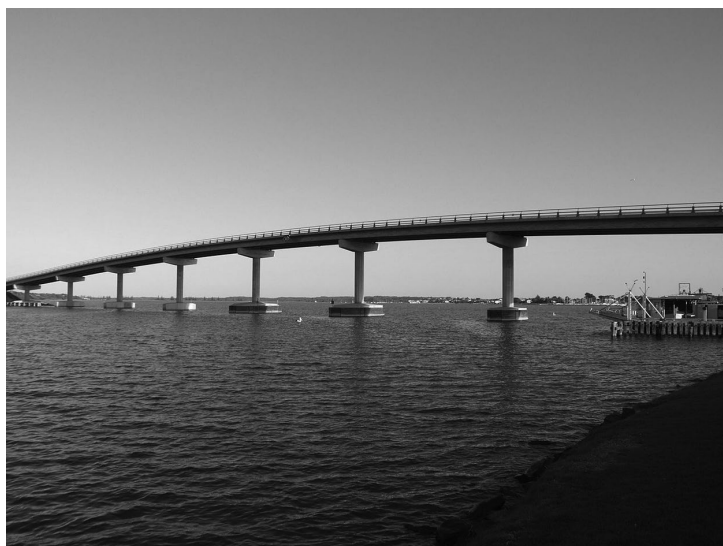
Figure 5.5 The Hindmarsh-Goolwa Bridge.
