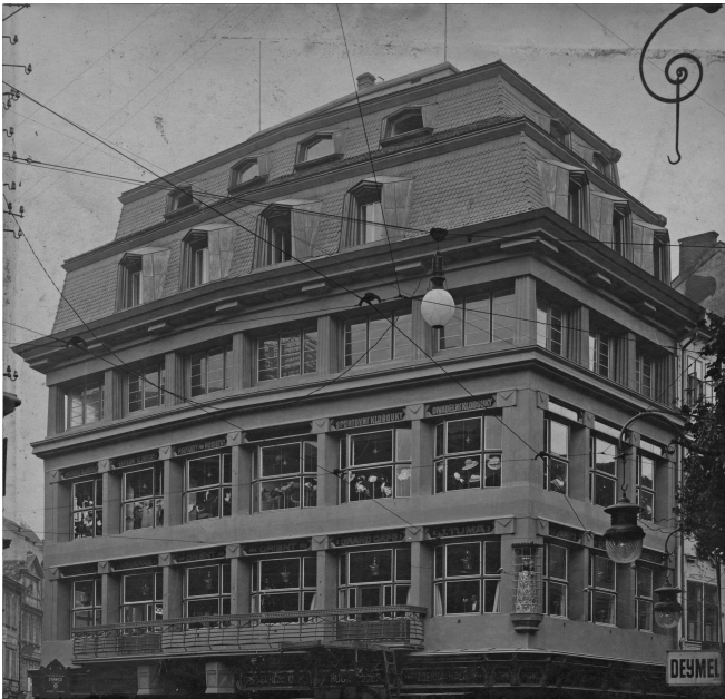
Figure 1.2 Josef Gočár, The House of the Black Madonna, Prague. Štenc studio, f. 14 Gočár. National Technical Museum, Museum of Architecture and Civil Engineering, Prague.
