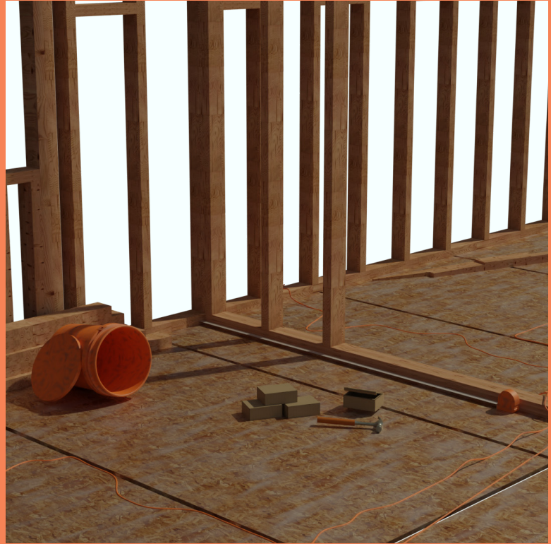
Install Blocking Boards
