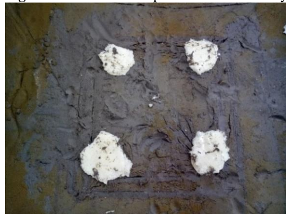
Figure 4. PU column after curing
