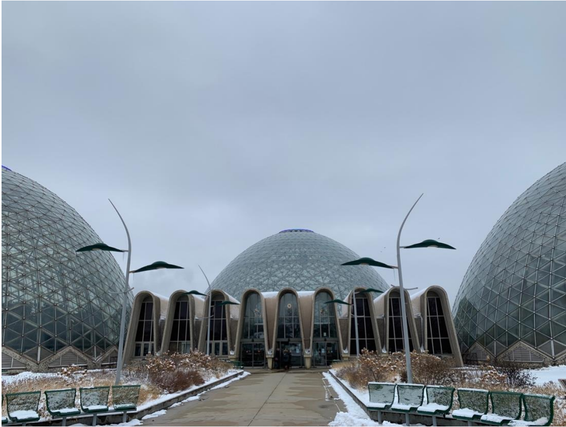
Concrete entrance elements at "The Domes," 64
