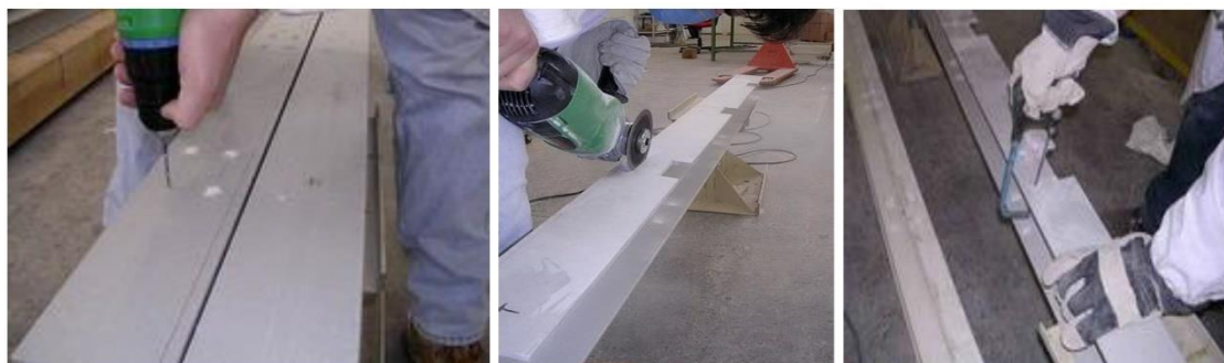
Figure 4. Notching procedure of the GFRP profiles.
