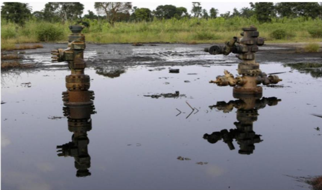
Figure 2.7 Leaks and spills of fracturing fluids in Bodo, Ogoniland Nigeria (source: Mohammed, 2012)
