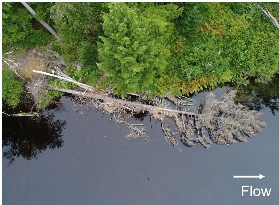
Figure 5. Aerial photographs (sUAS) of two sites on the Narraguagus River in Maine. (A) Post-assisted log structure (PALS) sites include multiple pieces of large wood fixed together to posts driven into the bed, while (B) griphoist (GH) sites include one or multiple trees pulled into the river from a nearby bank.
