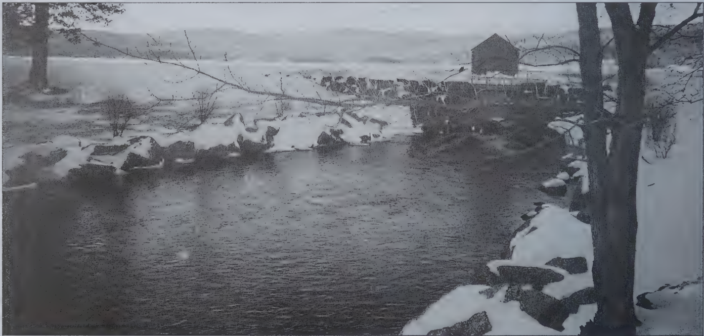
Elkins Dam, photo by Nadine Thomson
