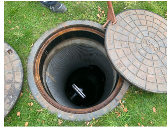
(b) Manhole (Ishøj, Denmark).
