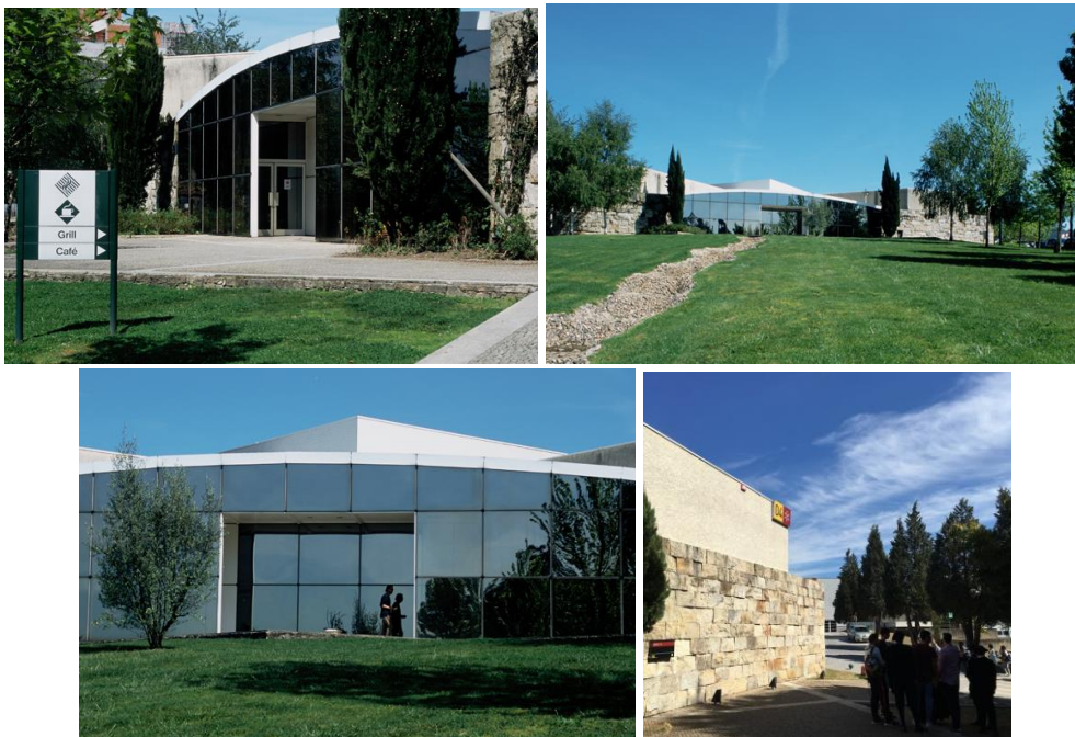
Figure 17: Photos of the Canteen building's exterior façades [69]
