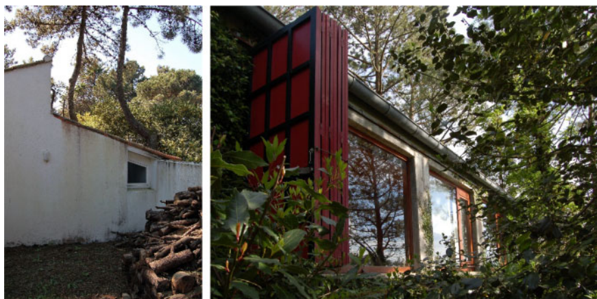
Figures 11, 12. Álvaro Siza, Alves Costa house (1964-71); Sergio Fernandes, Villa Alcina (1971-74). Photos by Eduardo Fernandes.
