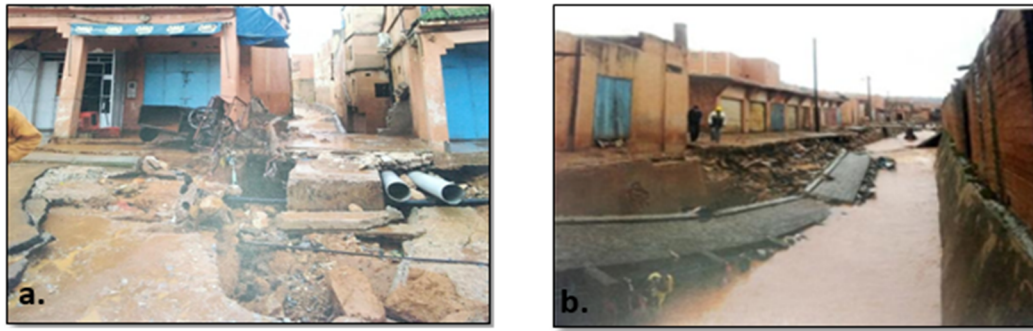
Figure 2. Damage to the infrastructure of the village of Lakhssas during the floods of November 2014. (a) Degradation of the National Road N°1; (b) Deterioration of the inter-provincial roads connecting Lakhssas village and Ifni city.
