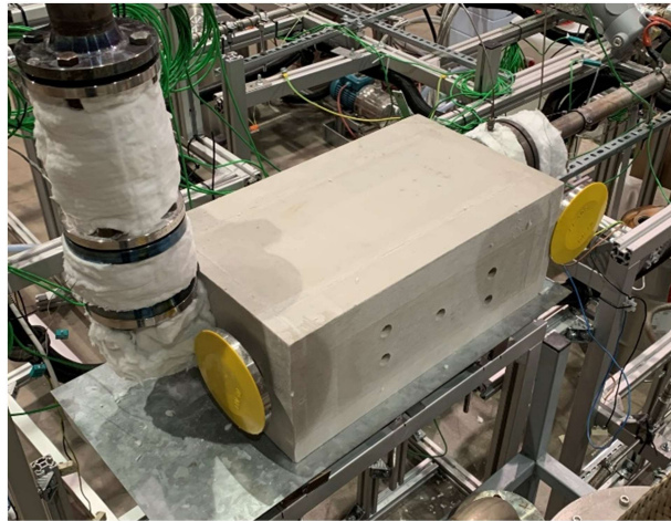
Figure 6. Close-up of the insulated 3D-PF-HEX during installation at the described test rig.
