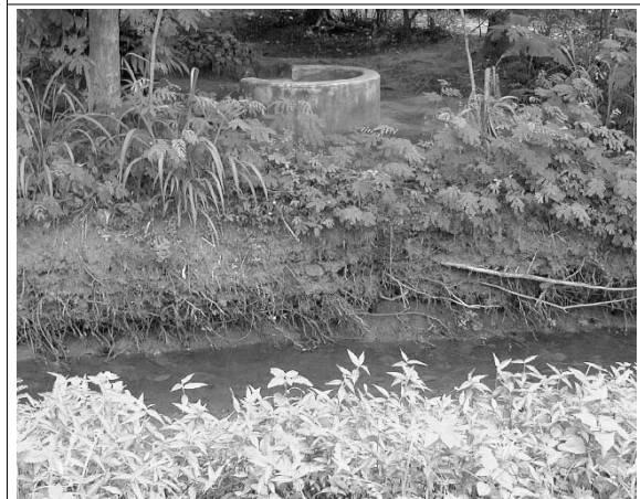
Fig. 2. Shallow well with protective concrete wall, located 3.7 m away from the earthen canal, Suriyawewa, Sri Lanka
