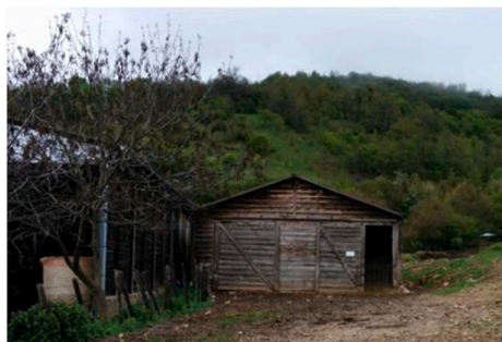
Fig. 5. Examples of emergency wooden shelters provided after 1997 earthquake to farmers of Serravalle di Chienti (MC) municipality (close to the epicentre in Colfiorito) (photos taken by one of the authors)
