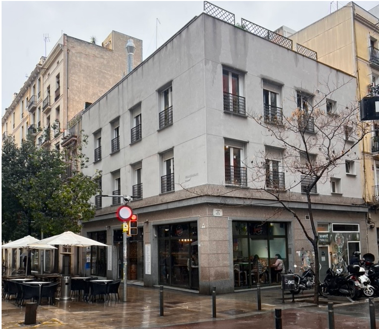
PICTURE OF BUILDING IN CURRENT STATE
