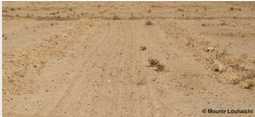
Figure 1. Soil surface scarification before rainy season (fall) to break soil crust
